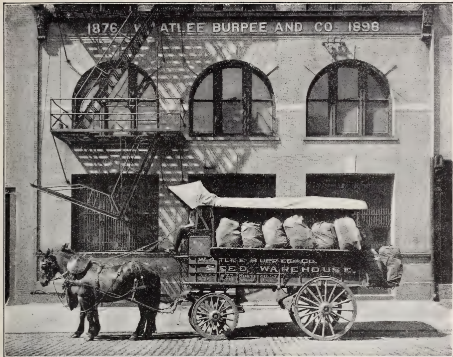
"READY FOR THE MAIL,"—at the York Avenue Frontage of the BURPEE BUILDING.
